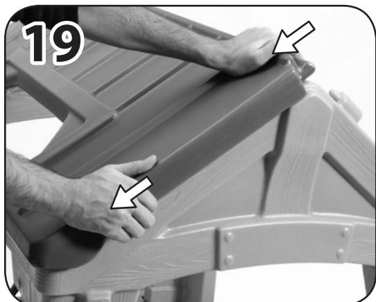
You will need a second person to hold the roof while securing to ensure there is a gap less than 4,76 mm (3/16") on both sides (21-24).
