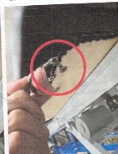
(Fix the hook with 2 15mm screws)
