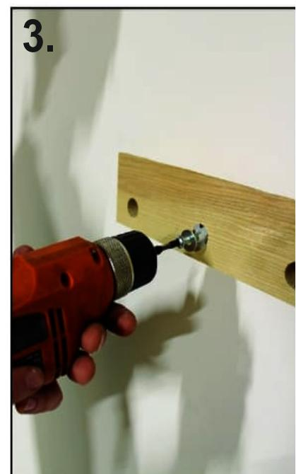
Secure the screws tight into the hole drilled in the wall with the help of drill
