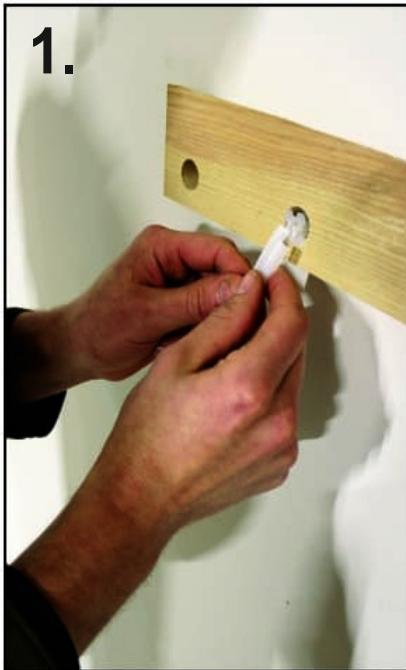
Insert the plastic dry wall anchor inside the hole drilled into the wall through the wooden support
