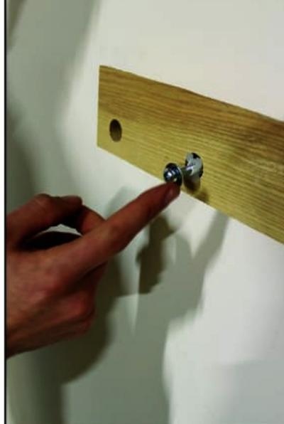
Thread the metal screw through the plastic washer until it threads till the wall
