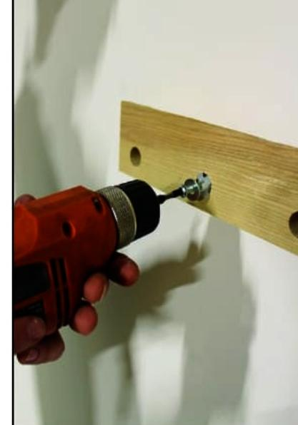
Secure the screws tight into the hole drilled in the wall with the help of drill
