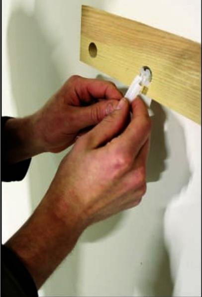
Insert the plastic dry wall anchor inside the hole drilled into the wall through the wooden support
