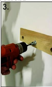
Secure the screws tight into the hole drilled in the wall with the help of drill
