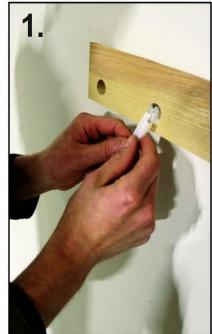
Insert the plastic dry wall anchor inside the hole drilled into the wall through the wooden support
